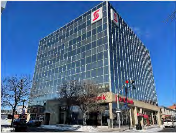
View from Corner of Cedar St & Durham St
