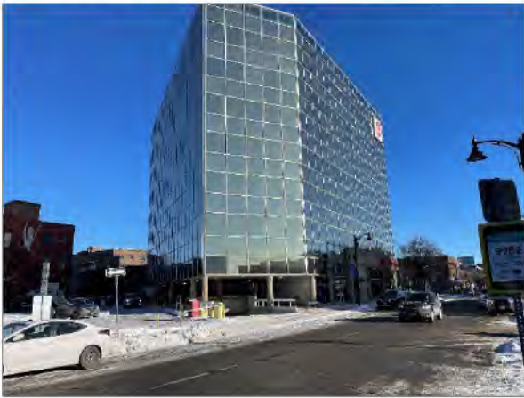
View Facing Northeast from Cedar St
