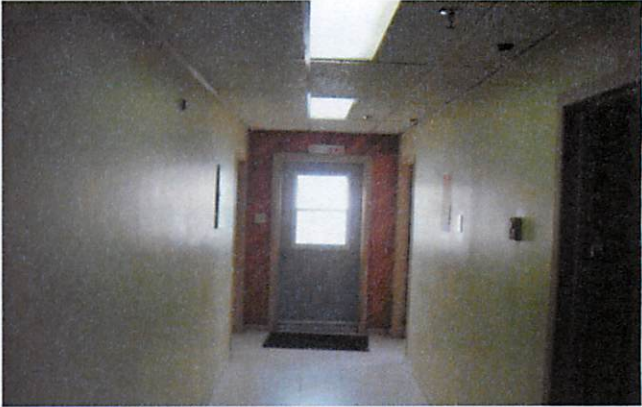
Interior office 2nd floor
